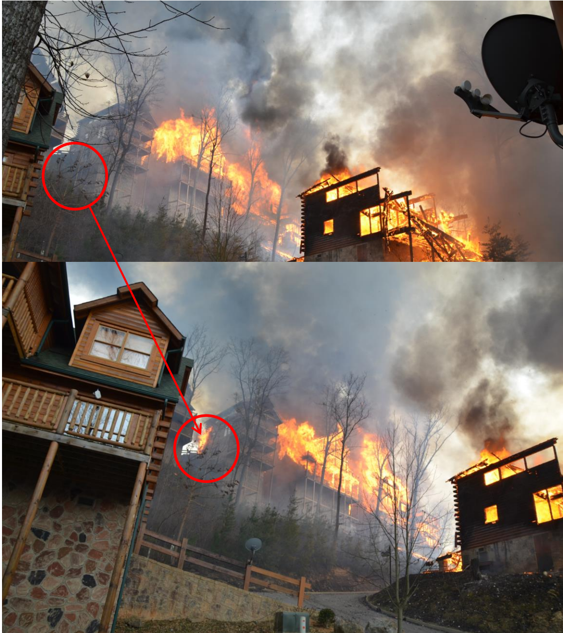
Figure 2. The first of two sequence figures taken by firefighters showing the growth of the fire at the front of a cabin. Note that in this figure and Figure 3, the circled areas are showing the same relative area. Photo credit: Chris Knutsen, Training Captain, Pigeon Forge Fire Department
