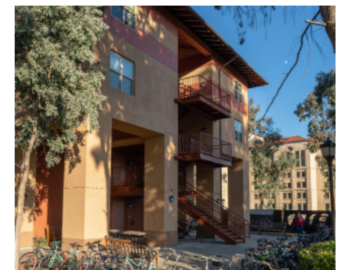
Escondido Village Studios, Exterior
